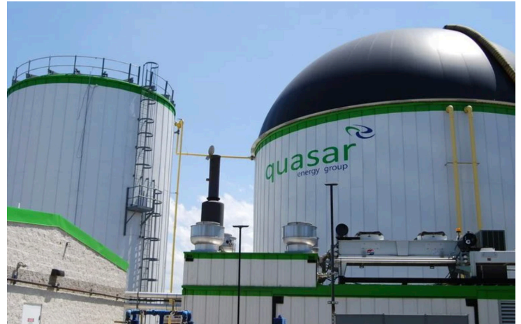
One of Quasar Energy Group’s anaerobic digesters in Cleveland’s Collinwood neighborhood.
